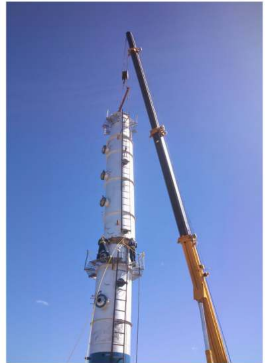
Erection Works of a Deodorizer
